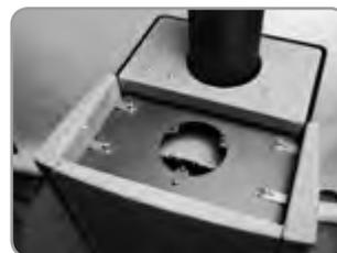
Now clean the stovepipe and the smoke flue and remove the residue with a vacuum cleaner. Return the elements to their initial positions and screw down the metal panel.
